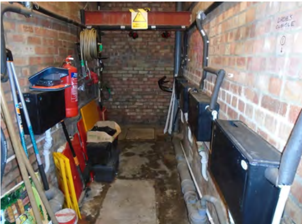
Internal View: Existing WC building
