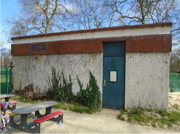
Existing WC building from the Playground
