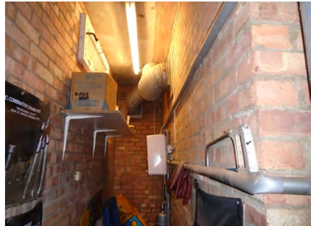
Internal View: Existing WC building
