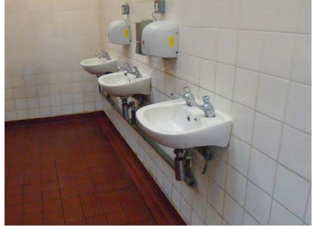
Existing WC building
